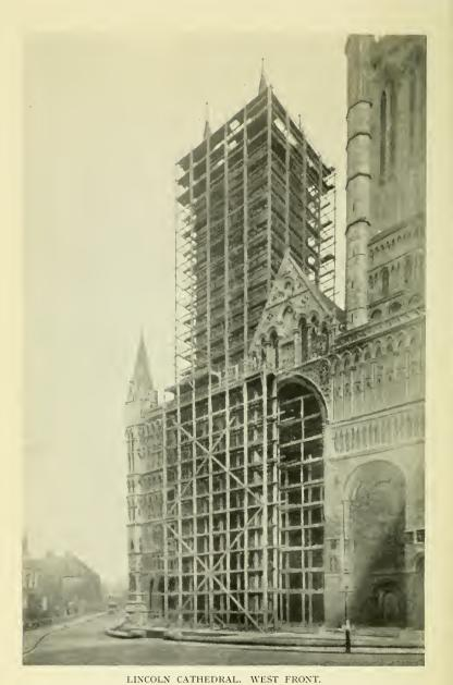
The great scaffold for repairing the North-West Tower, 215 ft. in height. When completed the scaffold will be moved to South-West Tower.
